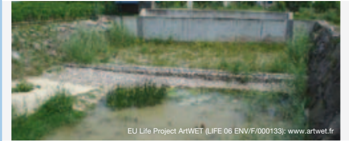
Water Retention Pond
